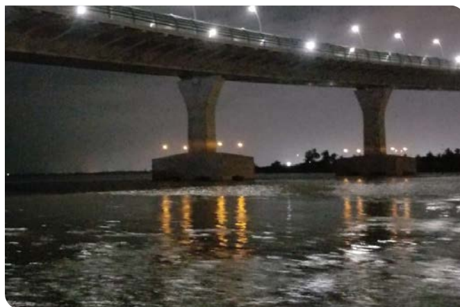
Two bridge abutments feature Sealite's SL-70 marine lanterns and flash in synchronization under the Pumarejo Bridge.
