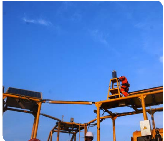
An Ecopetrol employee fits the SL-C510 Marine Lantern with integrated AIS to the top of the CALM buoy.
